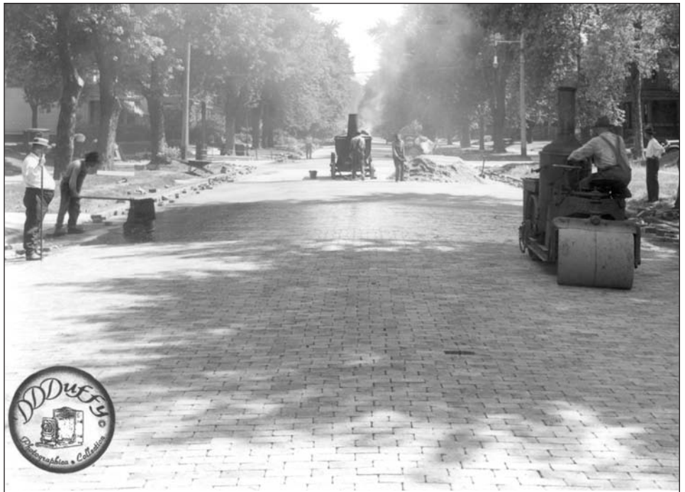
Road Contractors Steam Roller — circa 1930s
