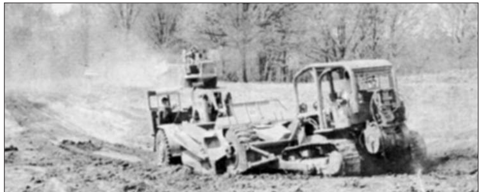
Tractor Push loads one of two scrapers on project.
