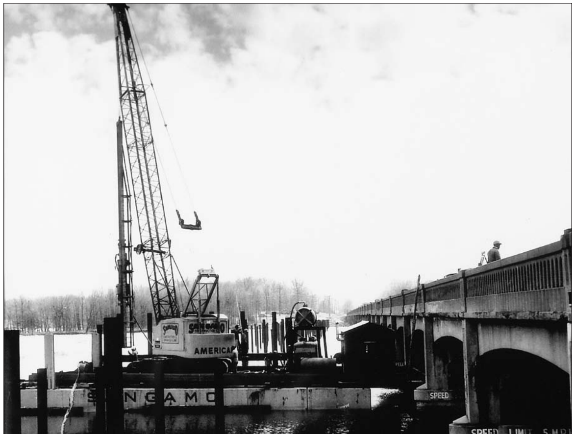
Sangamo Construction, Lake Springfield Bridge — 1968 Brother Glenn Albers operating crane
