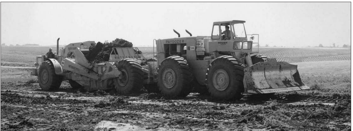
Lake Sangchris — 1955 Barrey Construction — Brother Robert Mathon operating a Paydozer
