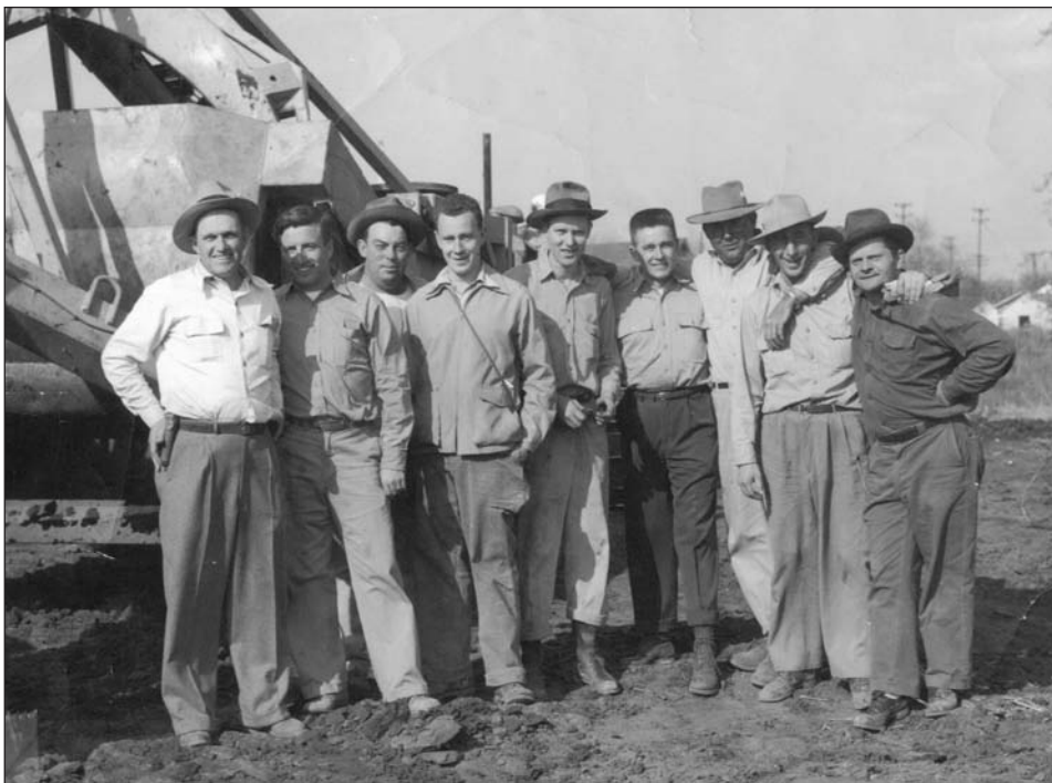
Building Jaycee Park
