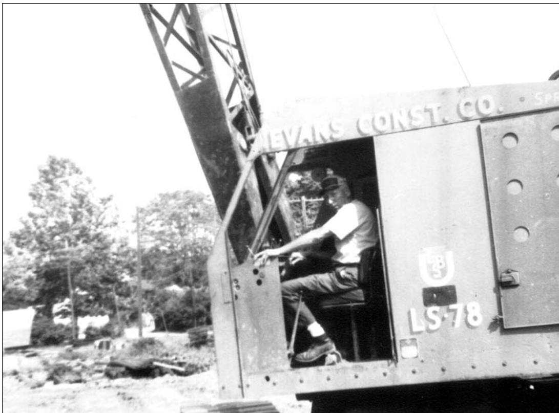
Evans Construction Company crane — circa 1960s Pete Ruzic is operator.
